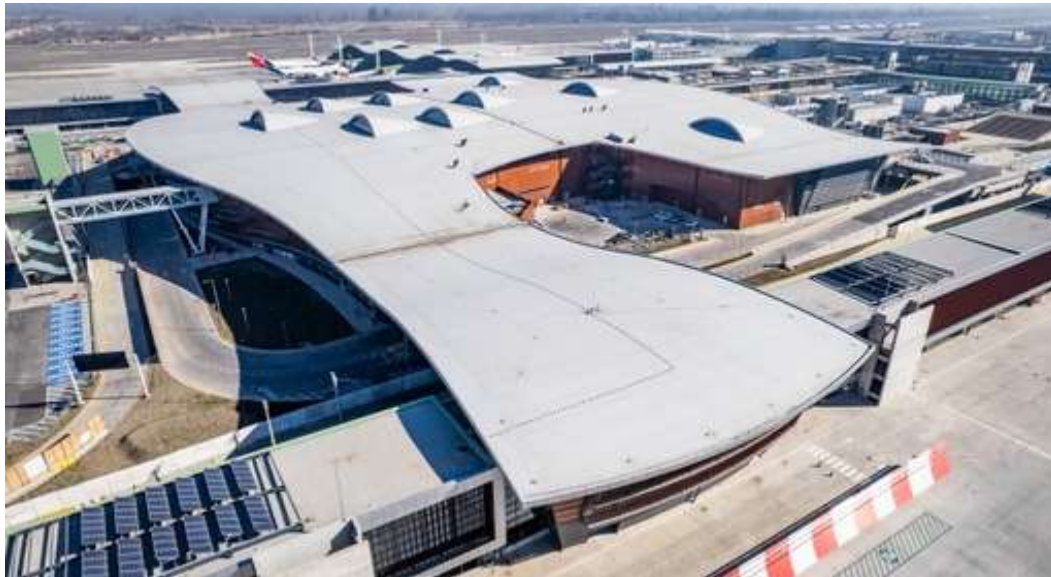
Figure 6.8 Arturo-Merito Benítez International Airport infrastructure development
